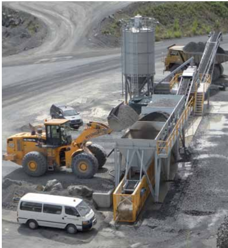
A loader loads various sized aggregates into feed bins. These are mixed, and cement and water added if required and then fed out into trucks.
